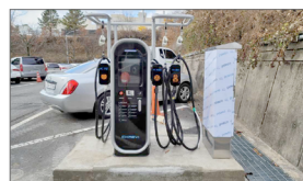
Installation of electric vehicle charger in front of main building
