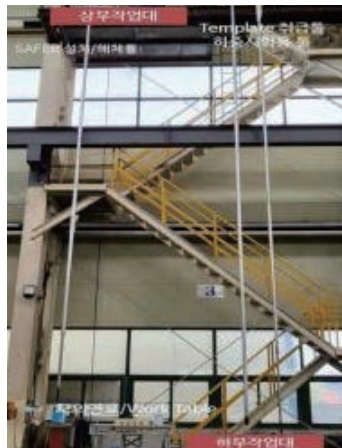
< Factory Acceptance Test >
